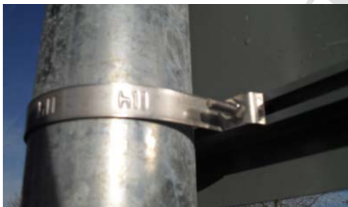
Stainless steel 114mm clip fitted around galvanised posts and into Rennicks stiffening channel.
